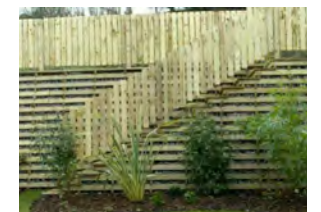
Timber cribblock wall.
