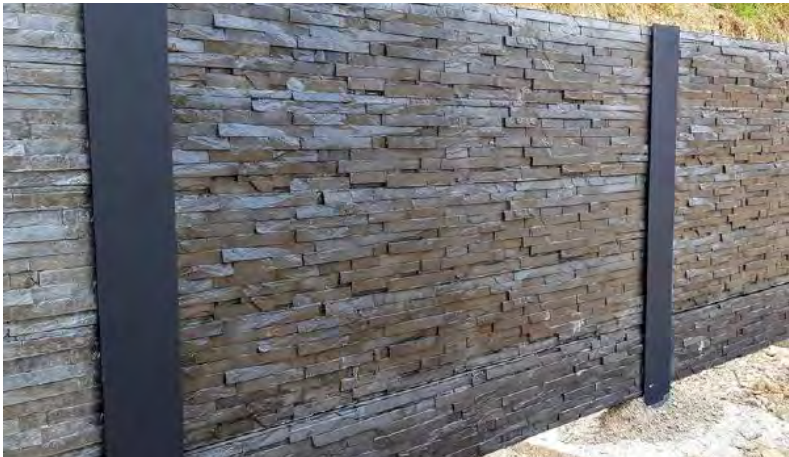
King post with textured concrete panel retaining wall
