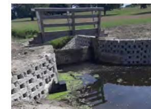
Aquacast outfall wall.
