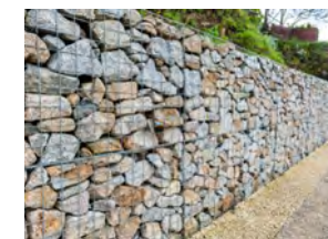
⌘ Stone finished face.
