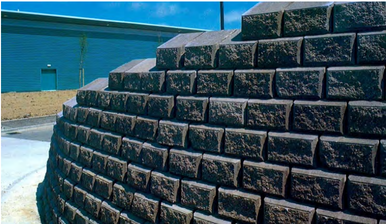
Chevloc retaining wall
