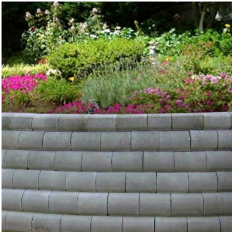
Porcupine garden retaining wall
