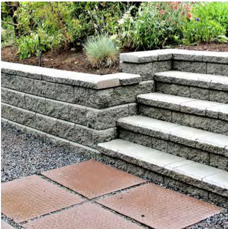
⤵ Keystone garden retaining wall
