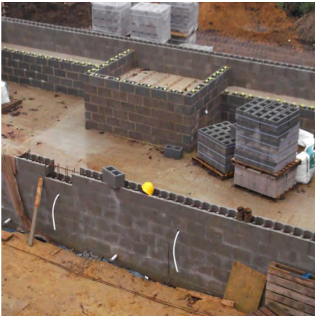
Stepoc basement retaining wall
