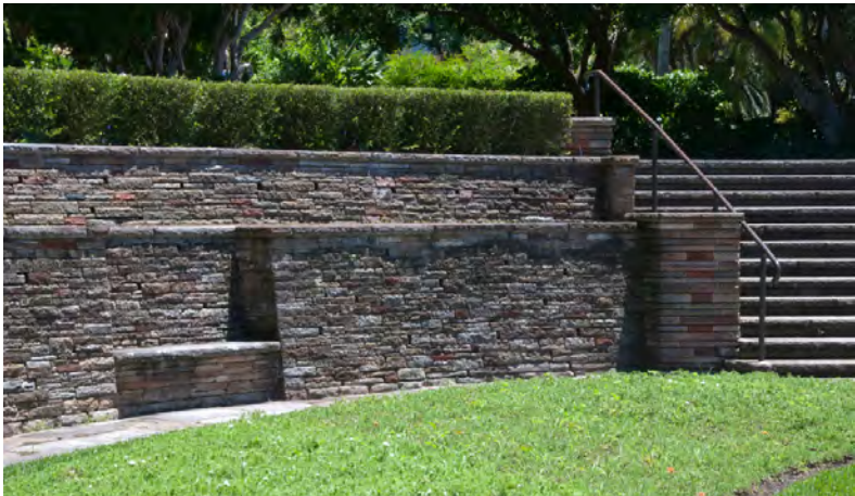
⤵ Stone clad masonry garden retaining wall
