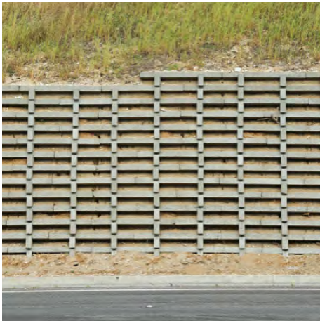
⤵ Concrete cribblock retaining wall
