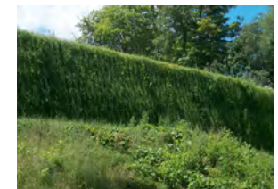
⚡ Geoweb® wall after seeding.
