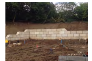
Inclined concrete block wall.
