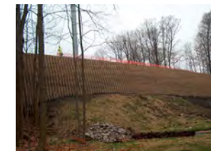
⚡ Geoweb® wall before seeding.
