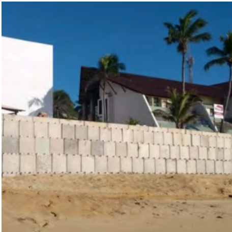
⤵ Gravity concrete block sea defense wall
