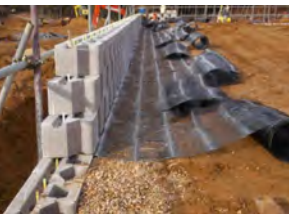
Keystone wall in construction.
