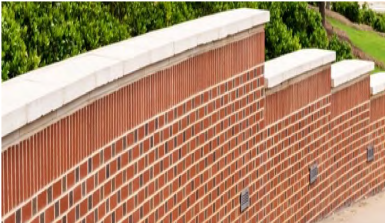
⤵ Brickwork masonry retaining wall
