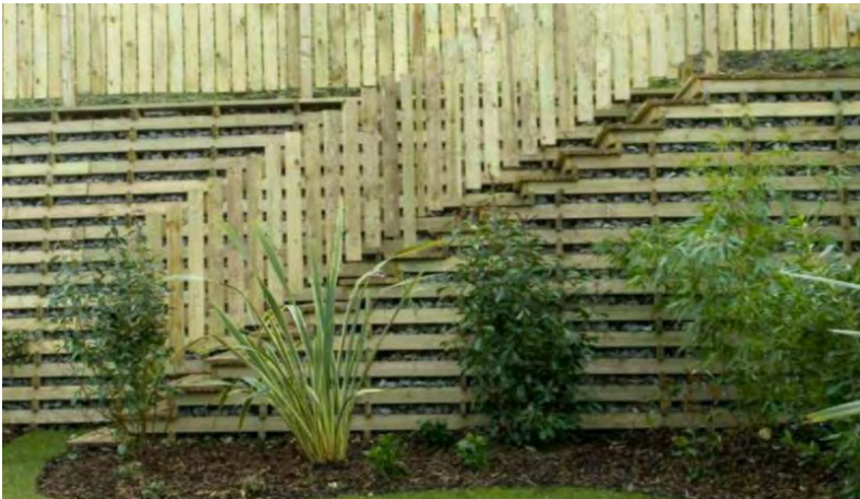
⤵ Timber cribblock retaining wall
