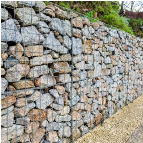
Stone filled gabion basket retaining wall
