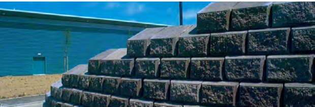
Stone finished face.
