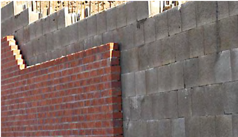
⤵ Brick cladded stepoc hollow block retaining wall
