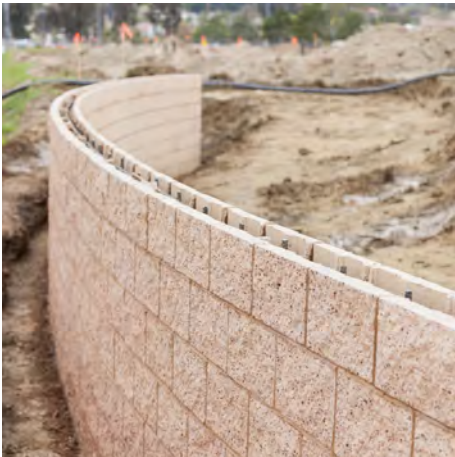
⤵ Concrete hollow block retaining wall
