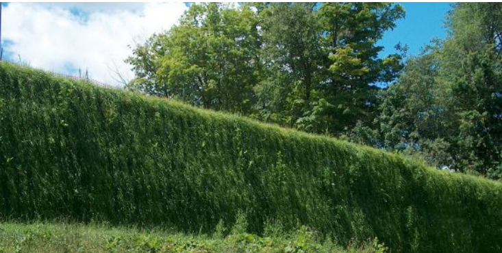
Geoweb retaining wall
