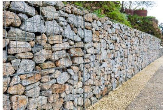
Gabion retaining wall
