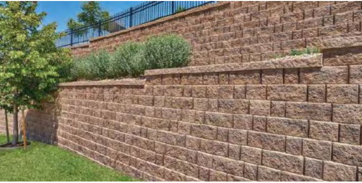
Keystone retaining wall
