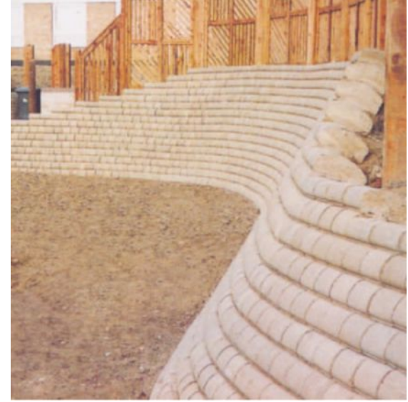
Porcupine retaining wall
