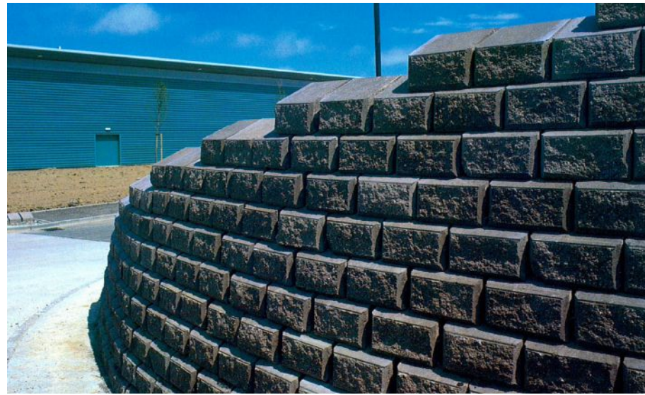
Chevloc retaining wall
