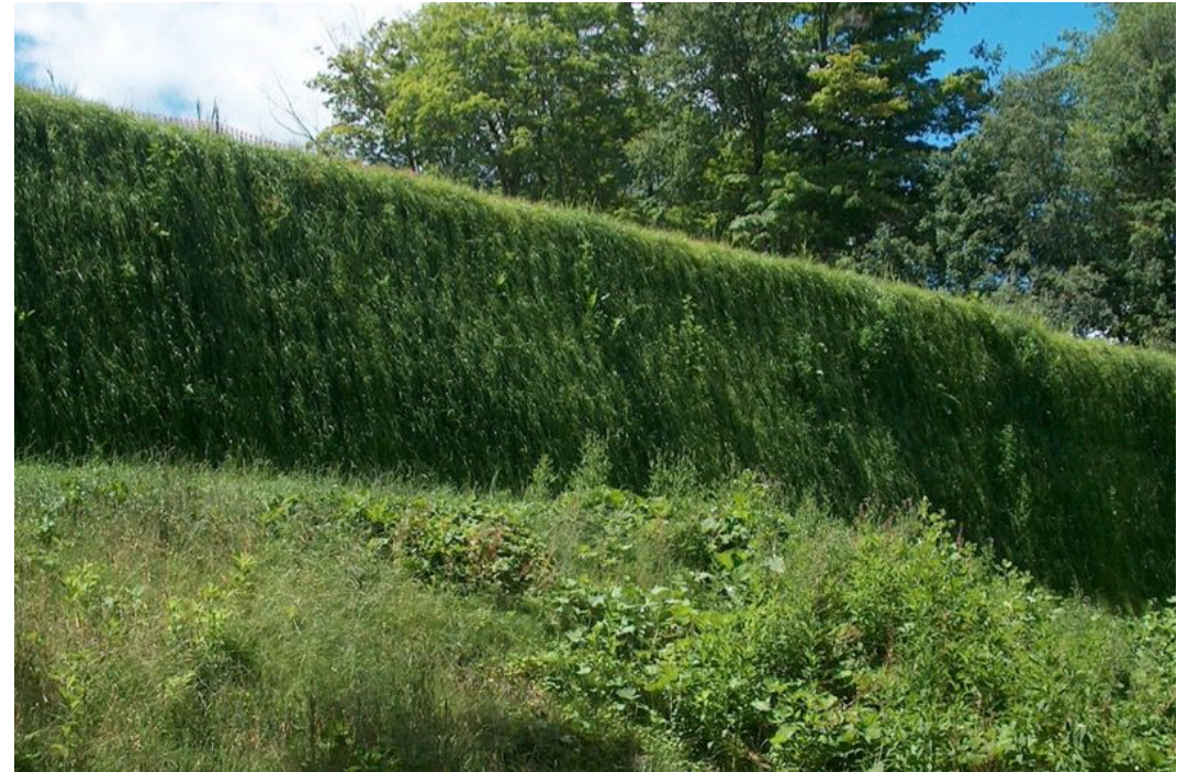
Geoweb wall after seeding
