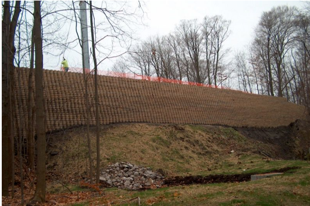
Geoweb wall before seeding
